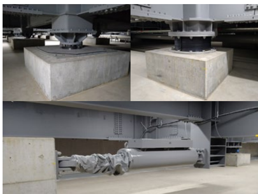
Hybrid seismic isolation structure
