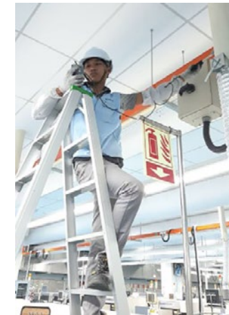
Eco Challenge Project at KL Technology Center of Sony EMCS (Malaysia)
