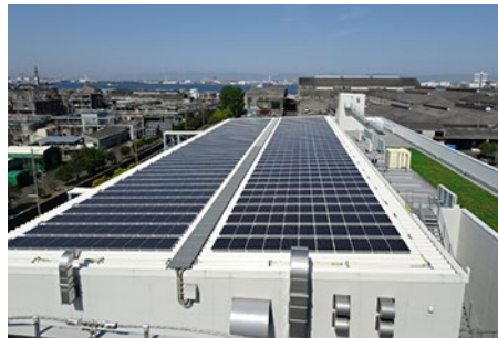
Rainwater collection system on roof of Green Cycle Corporation's plant No. 2
