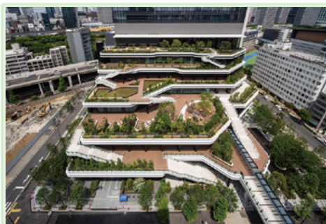
New Head Office Building: Tokyo Portcity Takeshiba Office Tower
