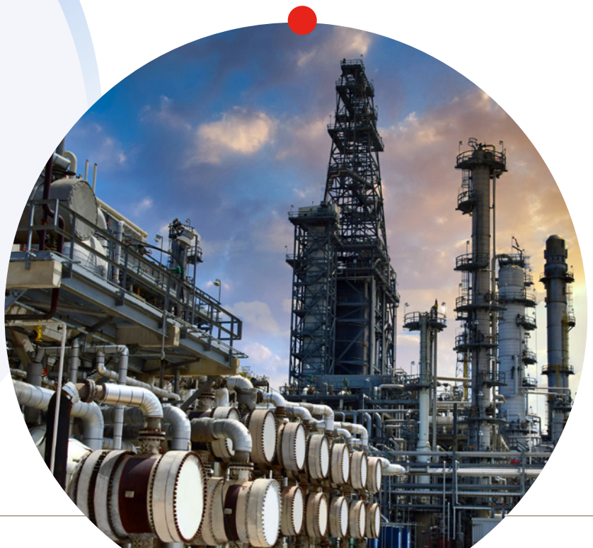
Borger Refinery BORGER, TX
