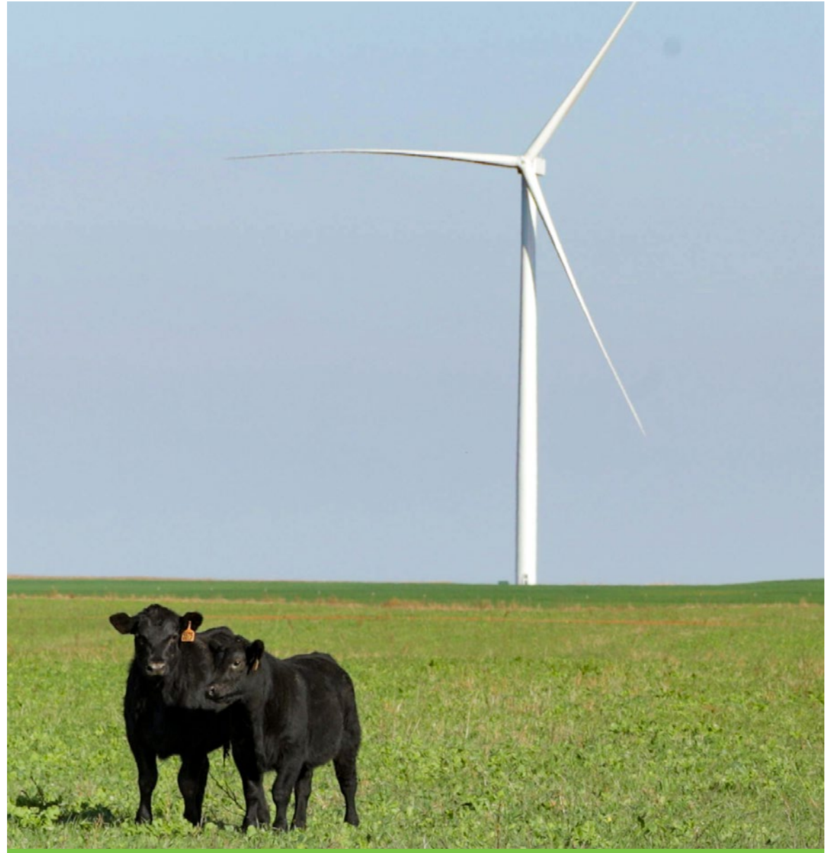
NextEra Energy Resources' Skeleton Creek Project located near Enid, Oklahoma.
