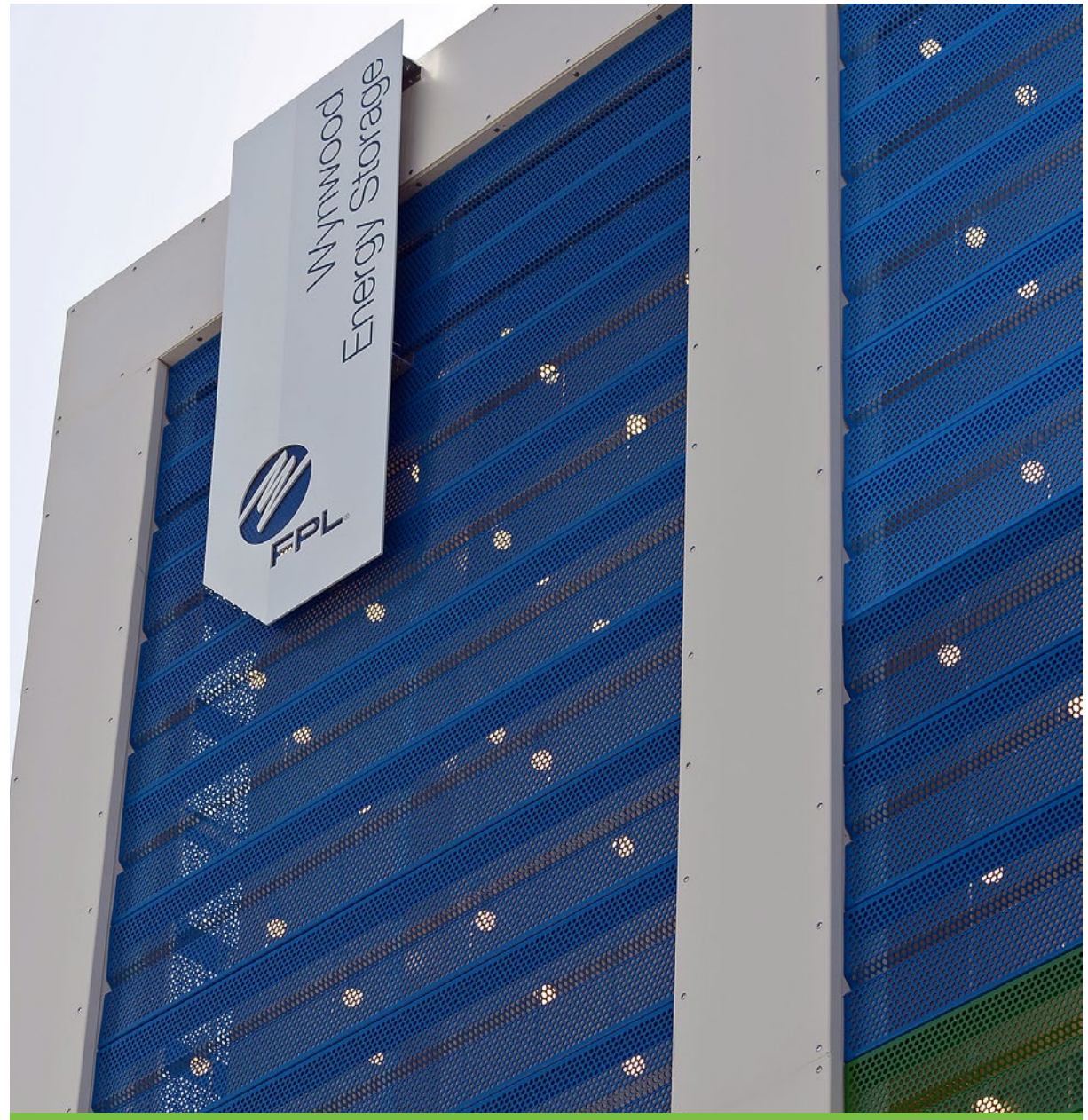
FPL Wynwood Energy Storage in Miami, Florida.
