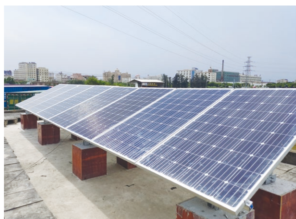
○ Fujian subsidiary piloted solar stacking with "solar energy + base station integrated energy cabinets"
