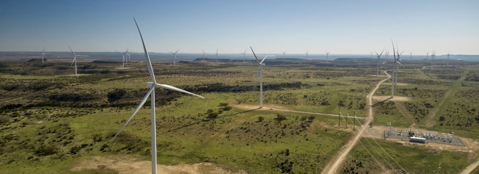
The Aviator Wind East project in Coke County, Texas became operational in 2020 and currently supports our operations in the region.
