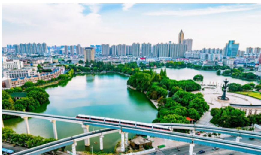
Anhui Branch supports the construction of the Wuhu Rail Transit Line 1. (Photo by Xu Jingran)
