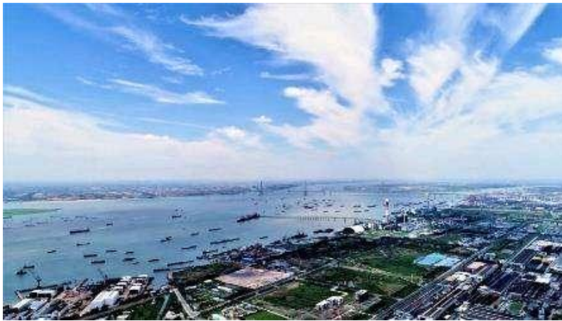
Chongchuan Sub-branch in Nantong, Jiangsu Province supports the supporting industrial cluster development of local shipping equipment. (Photo by Lu Nan)
